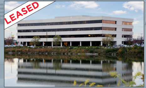
I-465 & 82nd Street Indianapolis, IN 1,100,000 sf
