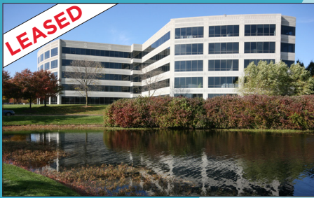
2 & 3 Woodfield Crossing Indianapolis, IN 386,000 sf
